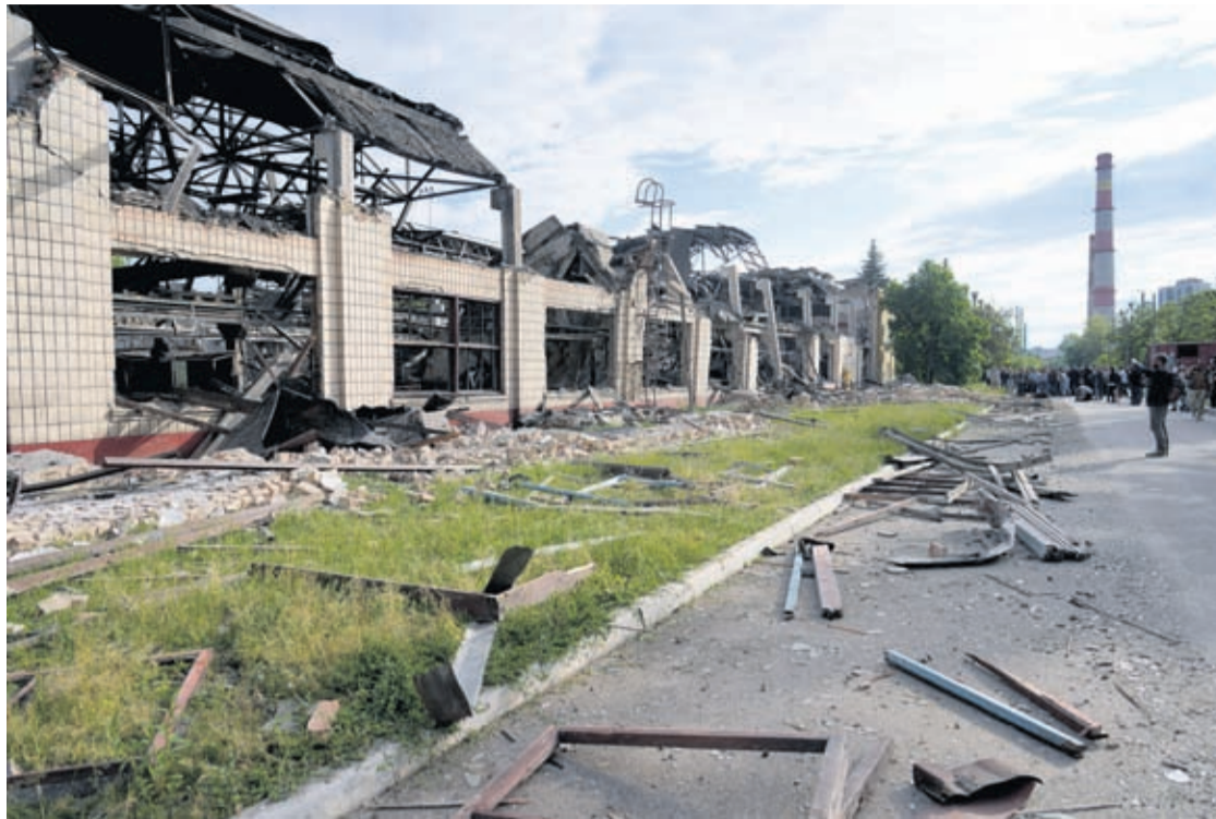
Wreckage lie along a street at a railway service facility hit by a Russian missile strike in Kyiv, Ukraine, Sunday, June 5, 2022.
